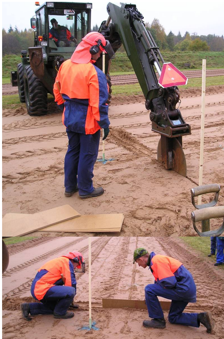
Figure A.3 – Proper fibreboard installation
